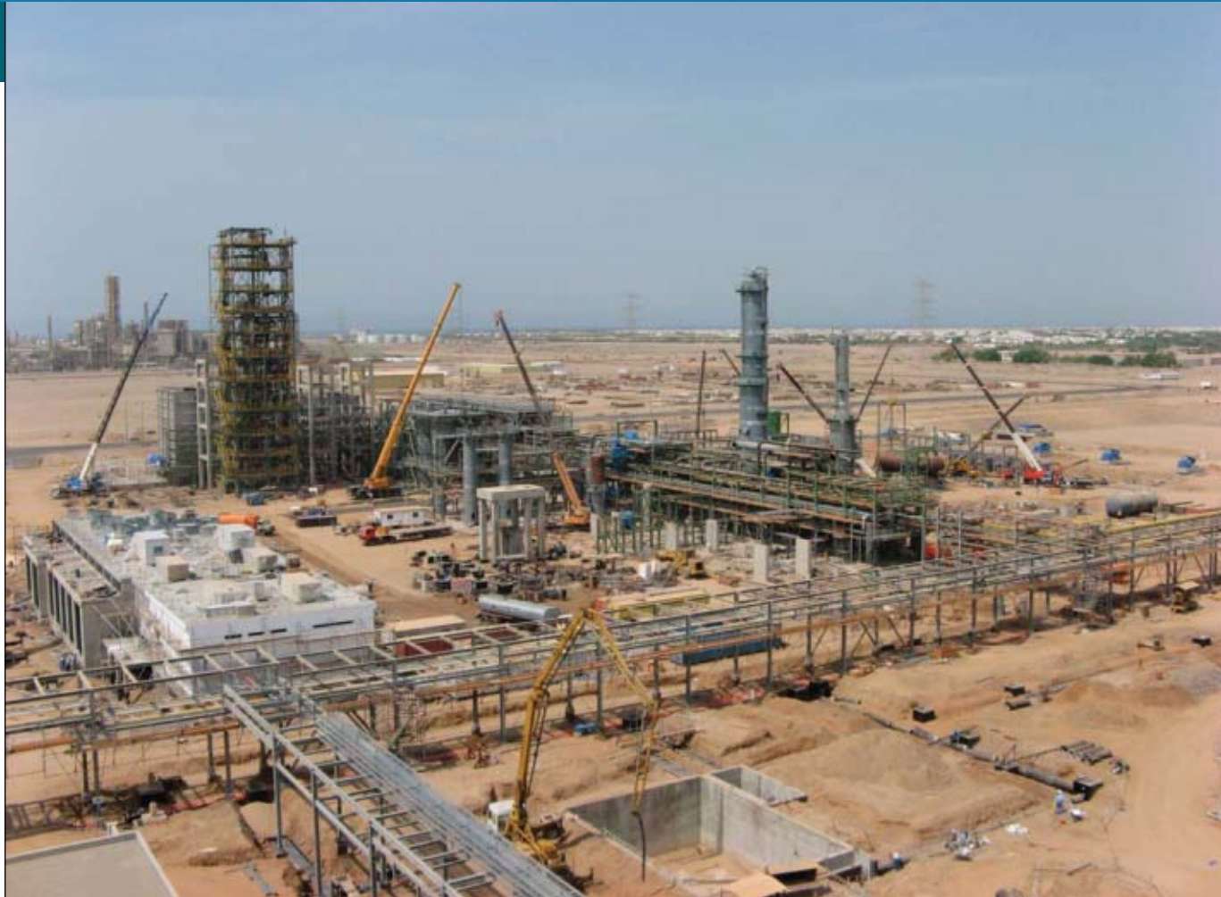
Construction progresses on the 400,000-tonne/year propylene plant in Yanbu by NatPet. The plant will begin operating by yearend 2007. Photo from Lurgi AG.
